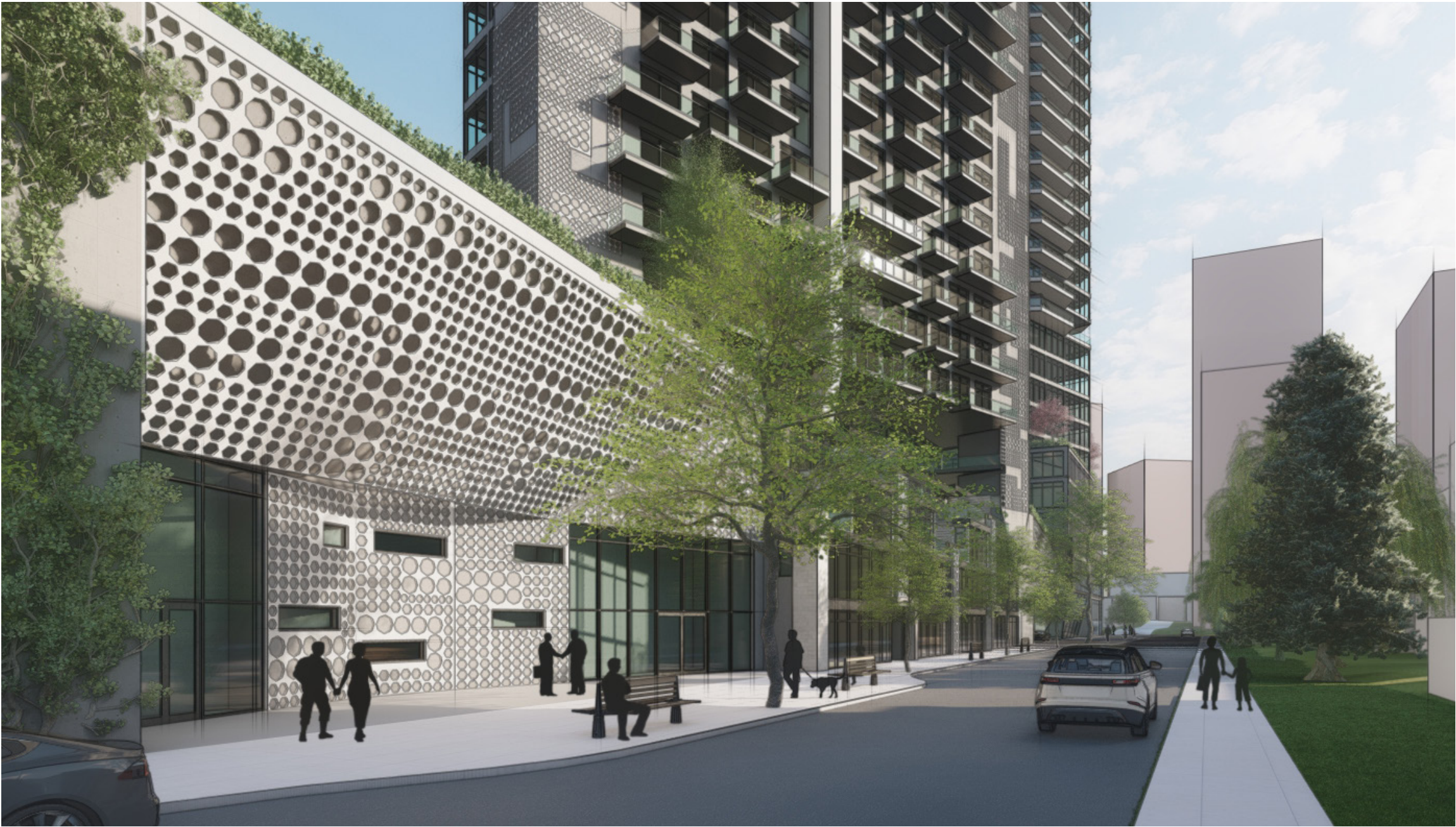
Perforated architectural screen concealing above-grade parking structure.
