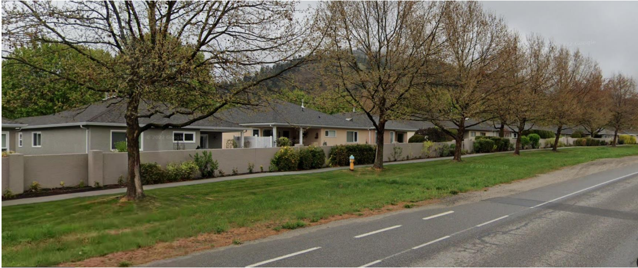
Fig. 2: Existing Strata Wall along Glenmore Drive.
