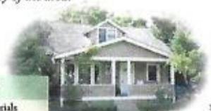
Stone House, built 1922, 1506 Abbott Street Built for Henry Stone in 1922, later associated with Abbott Society of Associated Grange of B.C., later the owner of Okanagan Ranch.
