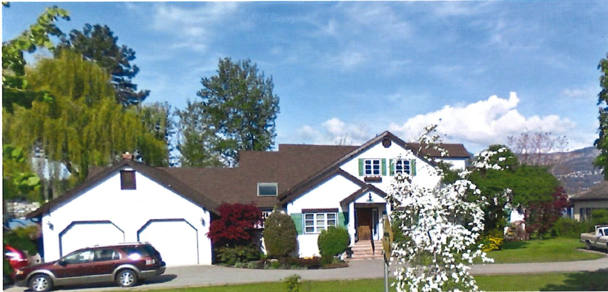
Above: current photographs of 2228 Abbott Street, constructed in the 1930s. Source: Google Streetview
