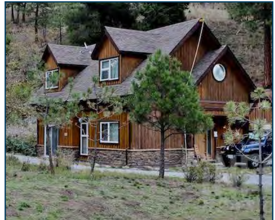
4. Caretakers Cabin Façade Renewal
