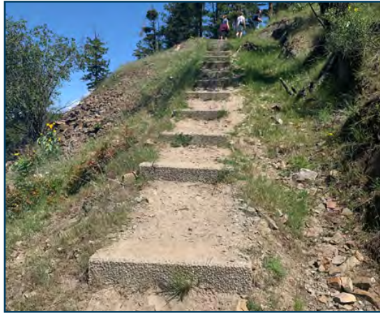
1. Ogoogo Trail – Step Replacement
