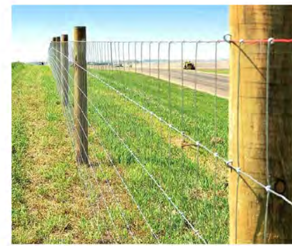
TYPICAL PASTURE POST & WIRE MESH FENCING
