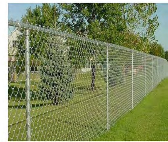
TYPICAL 6' HIGH CHAIN LINK FENCE
