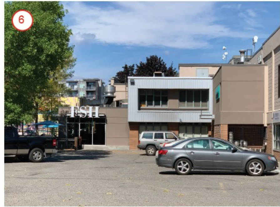
View of the current site condition - surface parking lot and lowrise commercial spaces from the south edge of the site facing north
