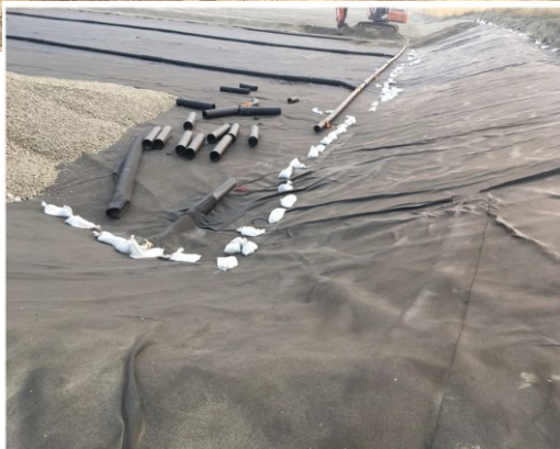
Photo #2: Area 2 leachate pipe being installed - Sep 17, 2020 12:00 AM
