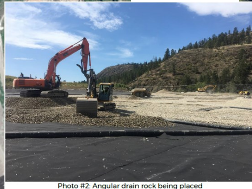
Photo #2: Angular drain rock being placed
