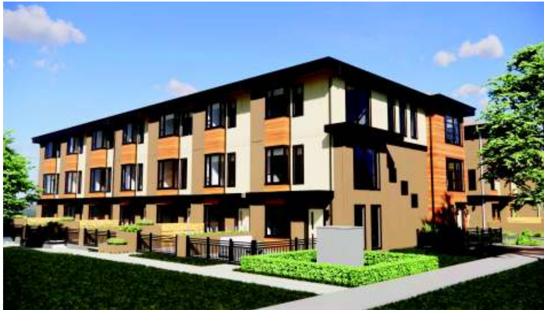
SOUTH EAST CORNER
