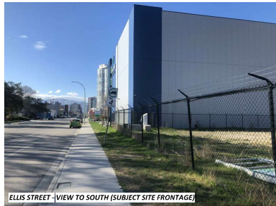
ELLIS STREET -VIEW TO SOUTH (SUBJECT SITE FRONTAGE)
