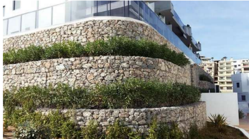
GABION RETAINING WALL WITH TERRACE PLANTING
