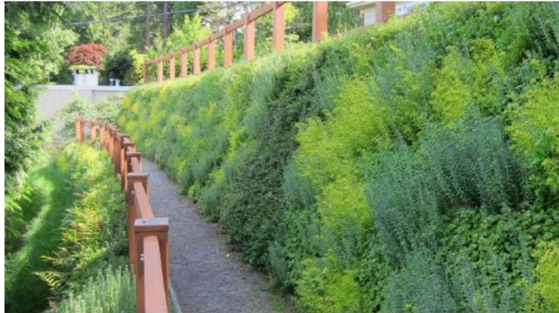
FLEX MSE RETAINING WALL
