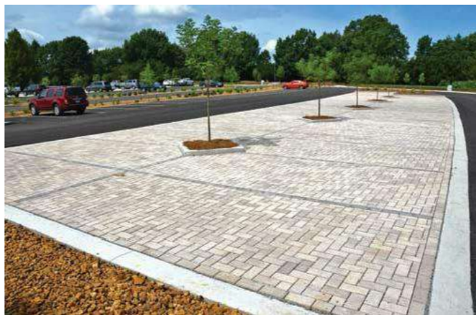
PERMEABLE PAVERS WITH FLUSH CURB
