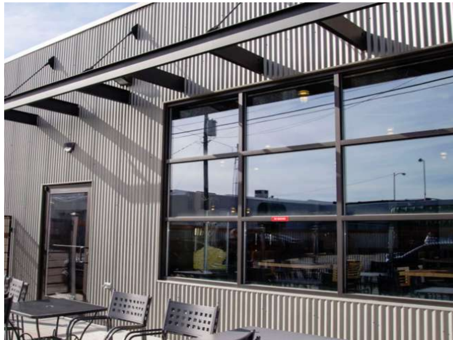
VERTICAL (#3) PROFILED METAL CLADDING - GALVANISED
