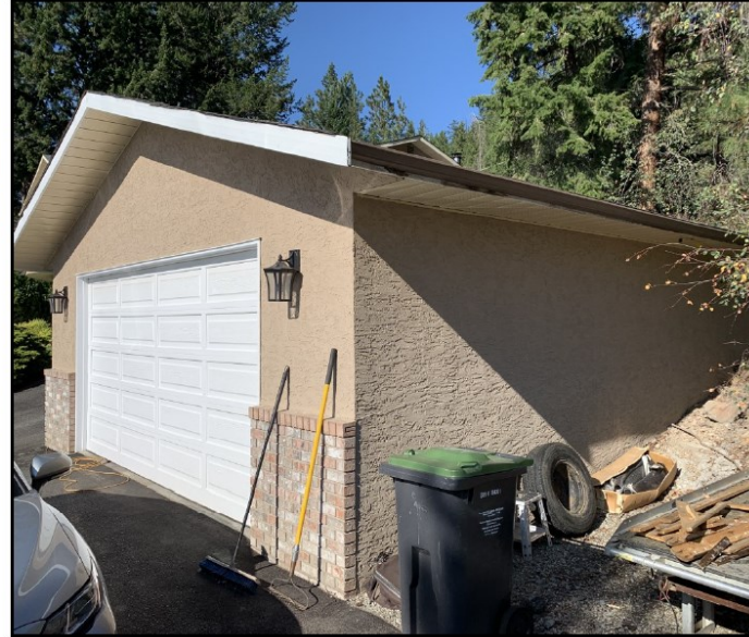
Southwest corner of garage
