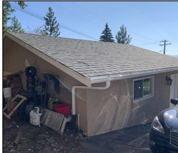
Rear of garage
