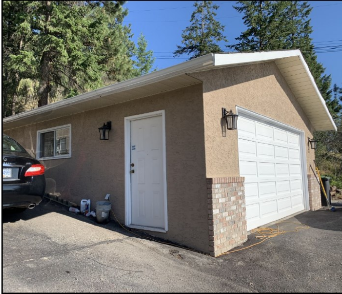
Northwest corner of garage
