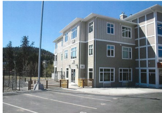
VIEW TO EXISTING ADJACENT EAST APARTMENT BUILDING
