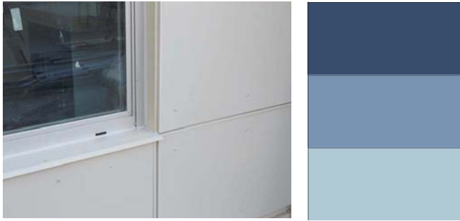
HARDIE REVEAL PANEL (SMOOTH) W/ PAINTED EXP. FASTENERS COLOUR PER MATERIAL LEGEND
