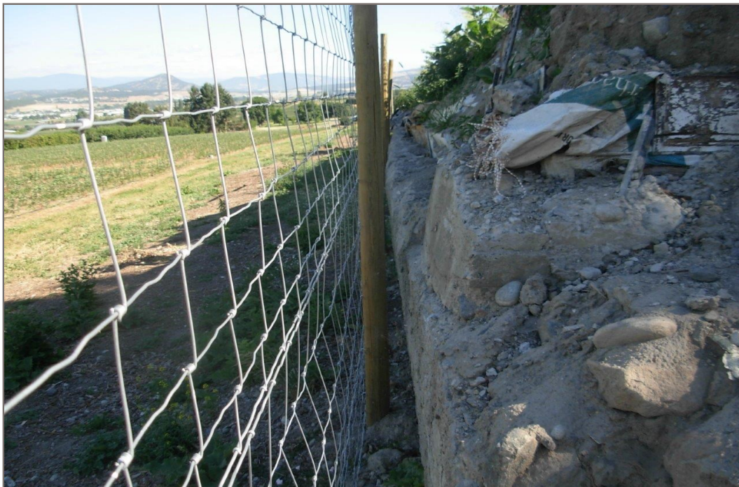
Photo 10: Lower wall. Approximately 0.80 m high wall. Looking to the north.
