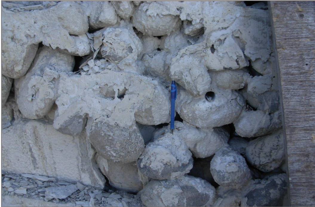
Photo 7: Upper wall gravel to boulder size rocks bounded with mortar.
