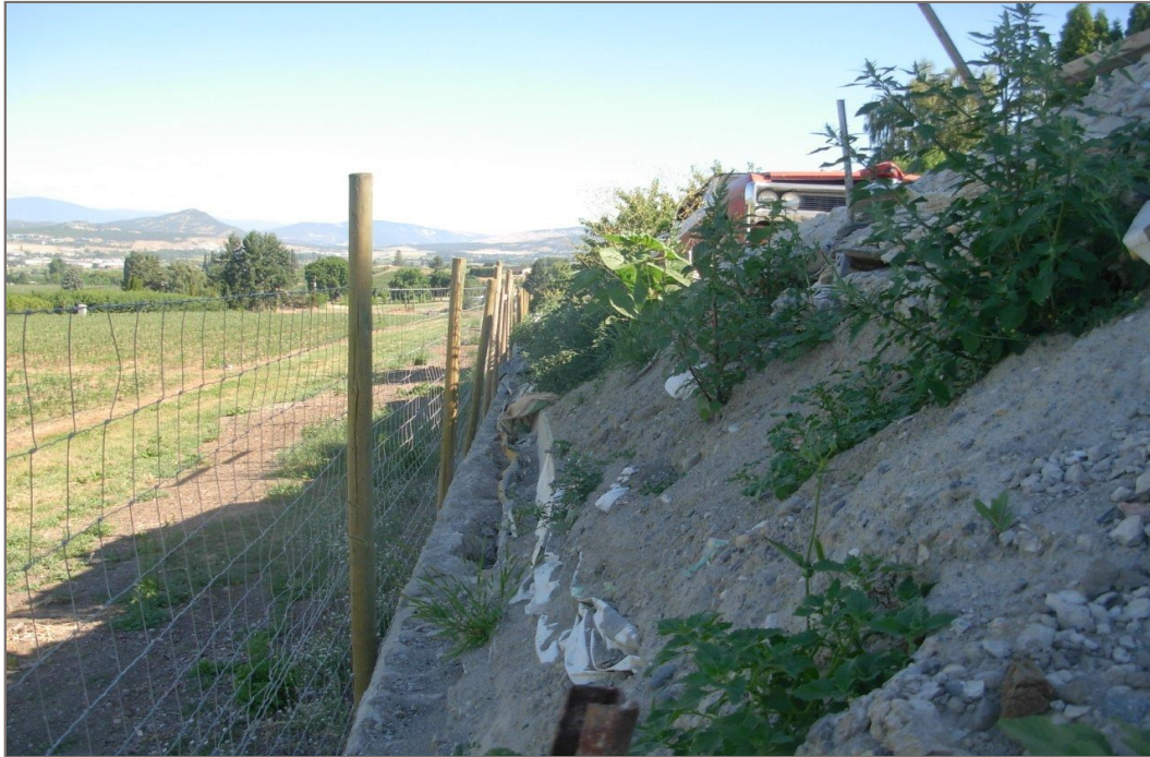
Photo 9: Lower wall and steep (~70°) 2.0 m high backslope.
