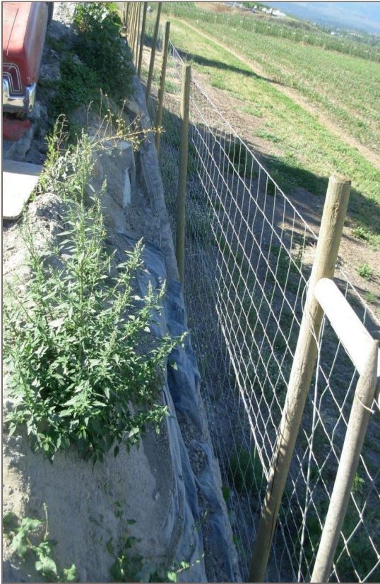
Photo 11: Lower wall looking south from top of backslope.
