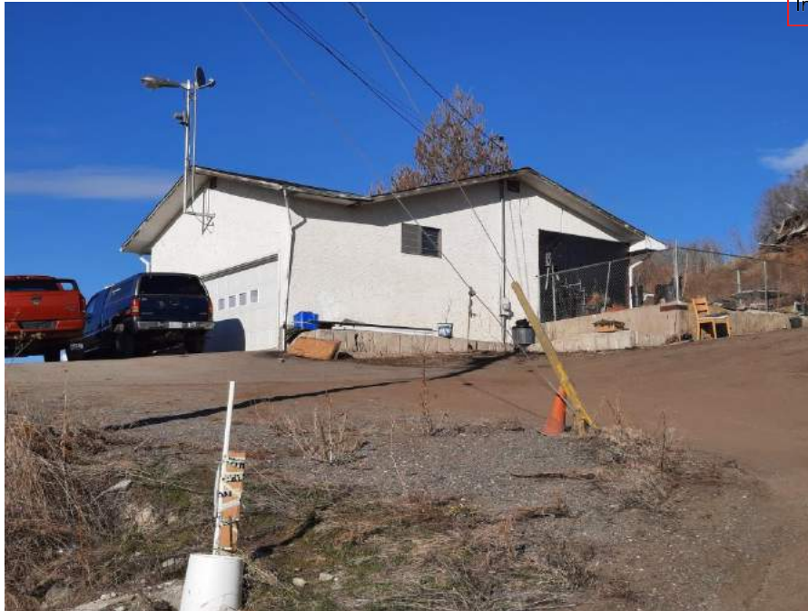
South side of existing house which is proposed for Farm Help & faces the proposed New House location
