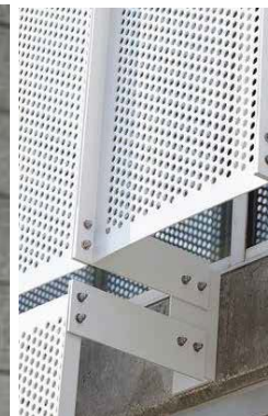
PERFORATED SCREEN ON EXISTING BLOCK
