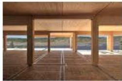
SAMPLE PHOTO CLT - Cross Laminated Timber Construction
