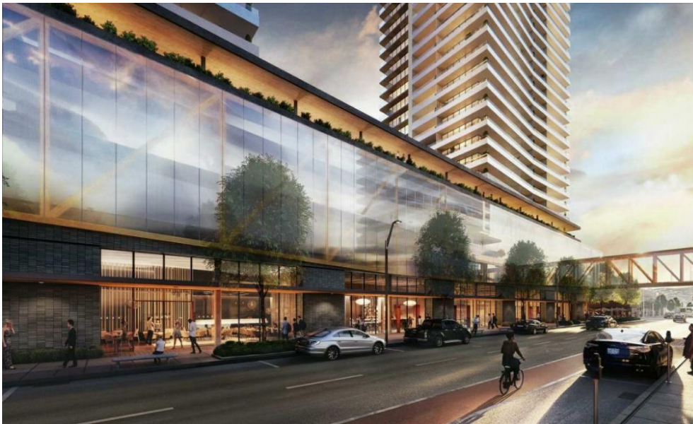
Fig 1.2 – Leon Avenue Elevation showing the polycarbonate screen and overall mass of the parking podium
