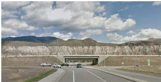
Highway 1 / Kokanee Way Interchange, Kamloops. Example of an interchange with the highway over the local road. (Source: Google Maps)
