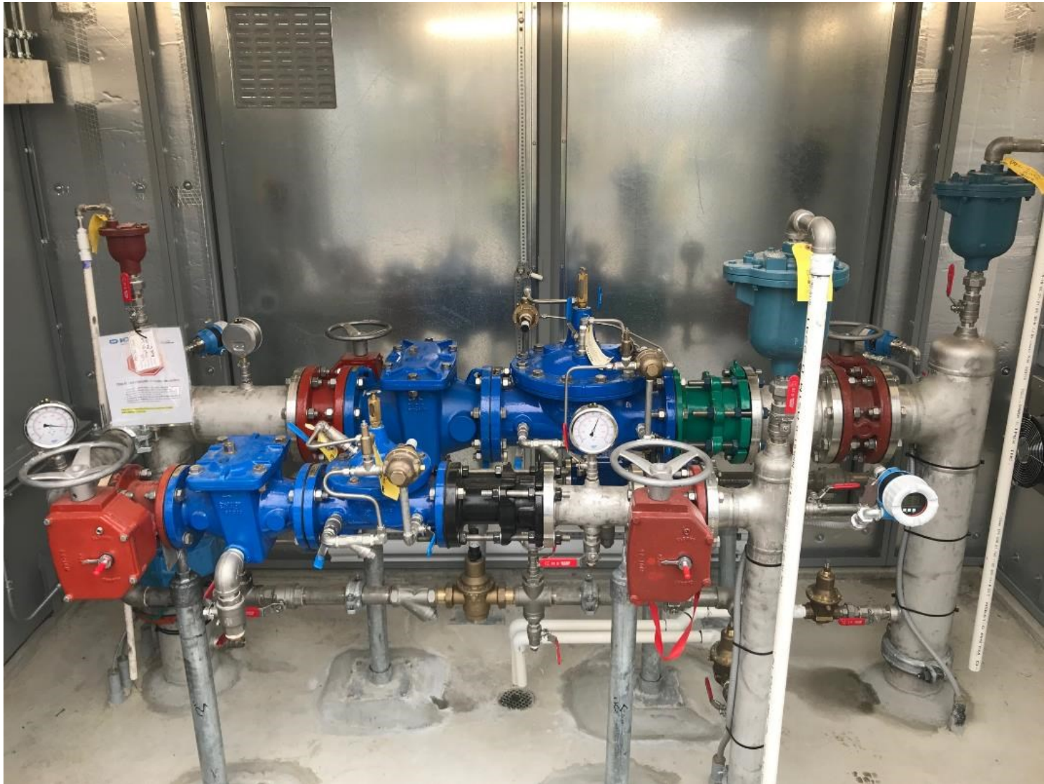
PRV serving dual pressure zones
