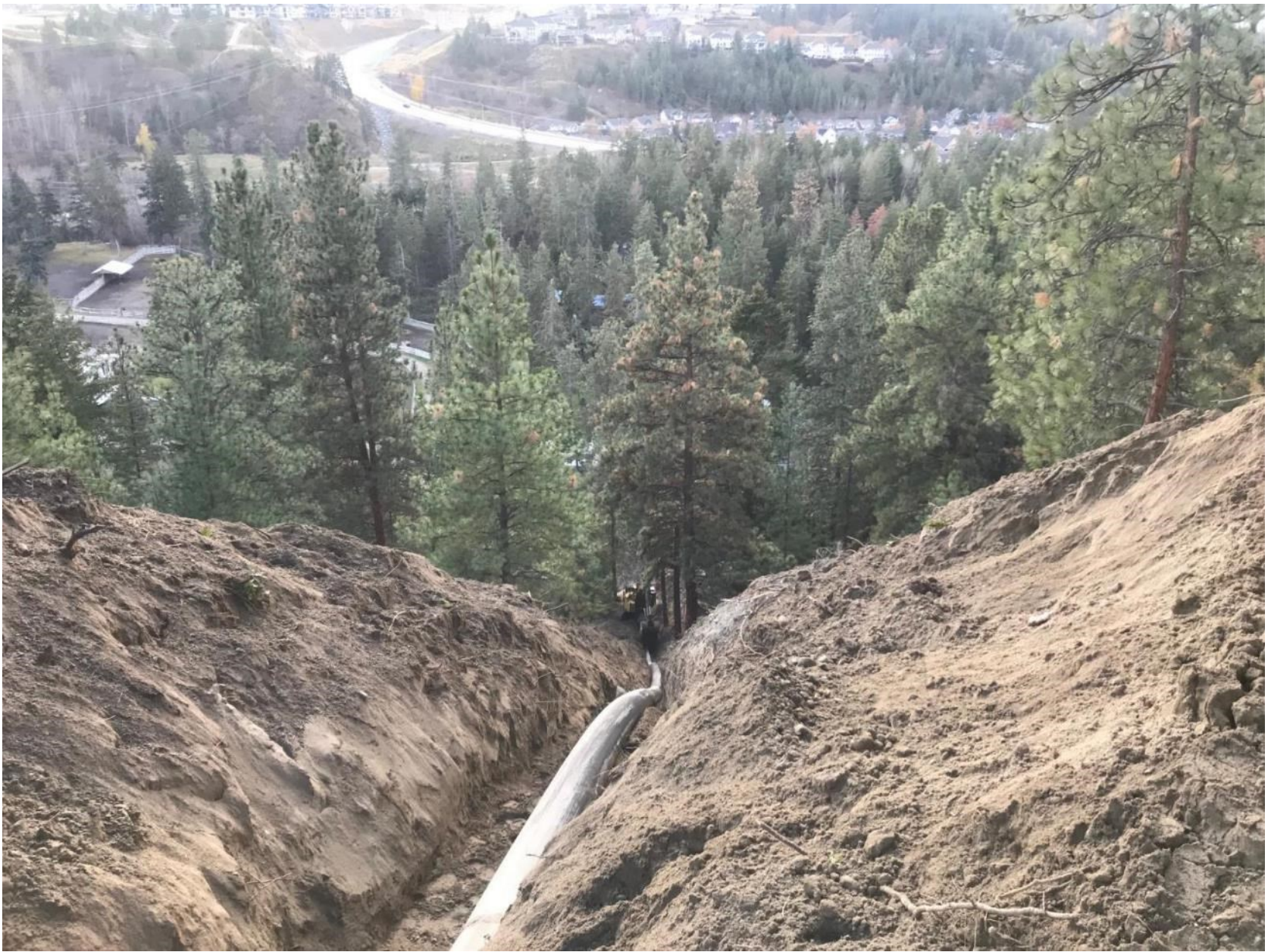
HDPE watermain used in challenging terrain
