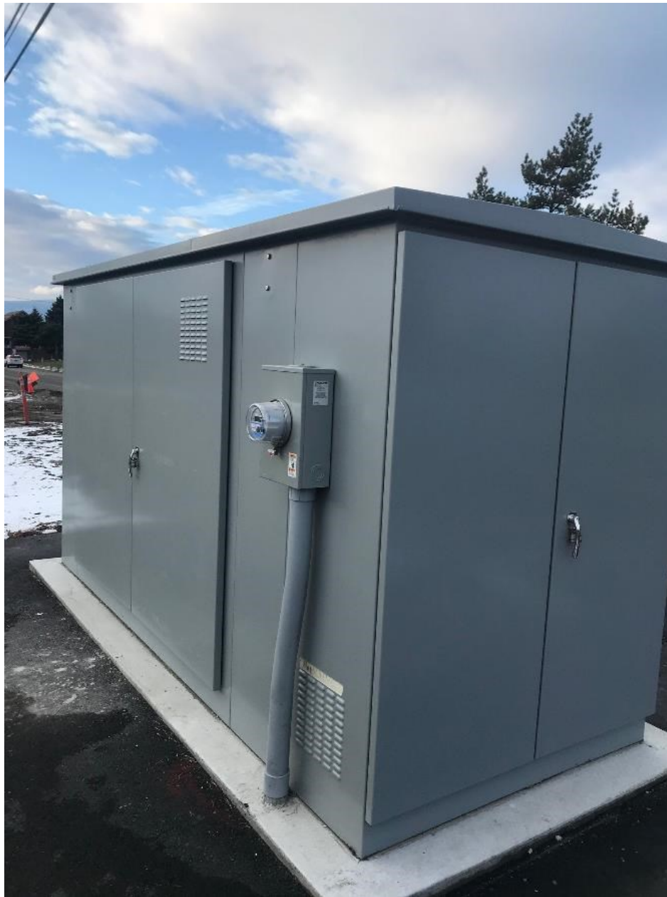
Pressure Relief Valve (PRV) in a kiosk
