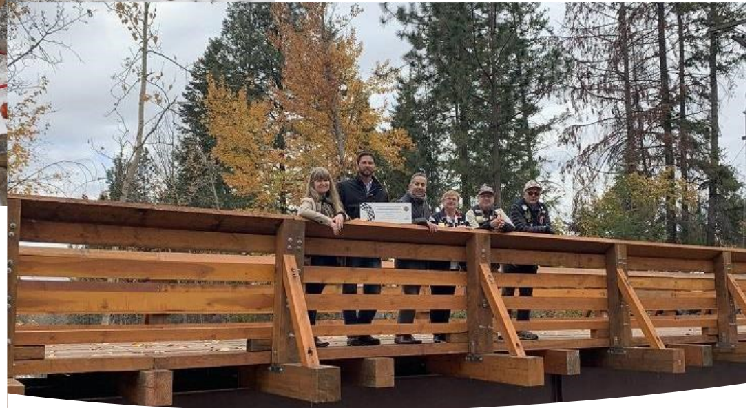
600mm trunk main across Bellevue Creek Pedestrian bridge was constructed to cross creek and improve pedestrian access
