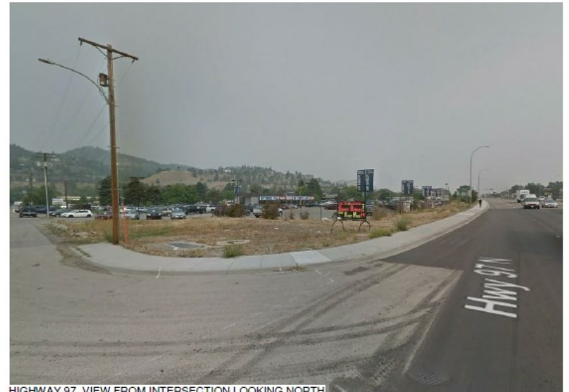
HIGHWAY 97, VIEW FROM INTERSECTION LOOKING NORTH
