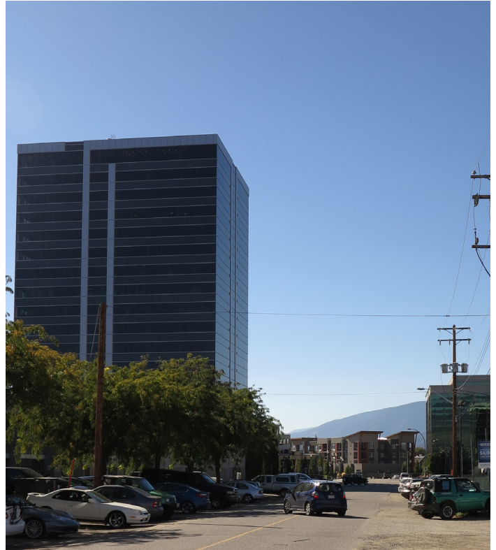
Lack of pedestrian infrastructure in Capri-Landmark
