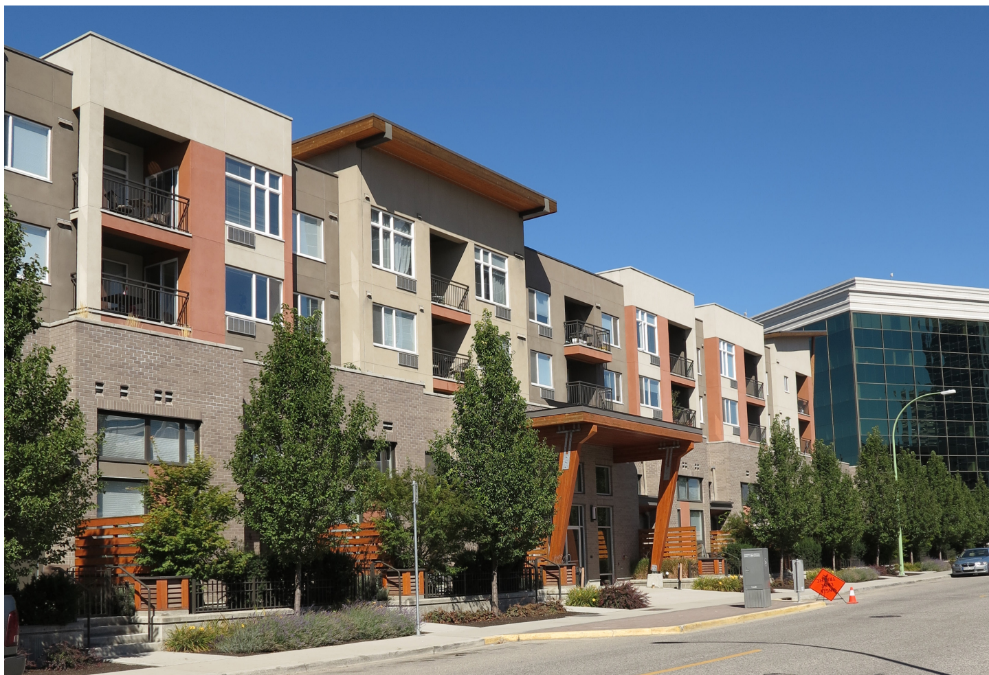
An example of a recent multi-family residential project (Mode) in the Capri-Landmark Urban Centre
