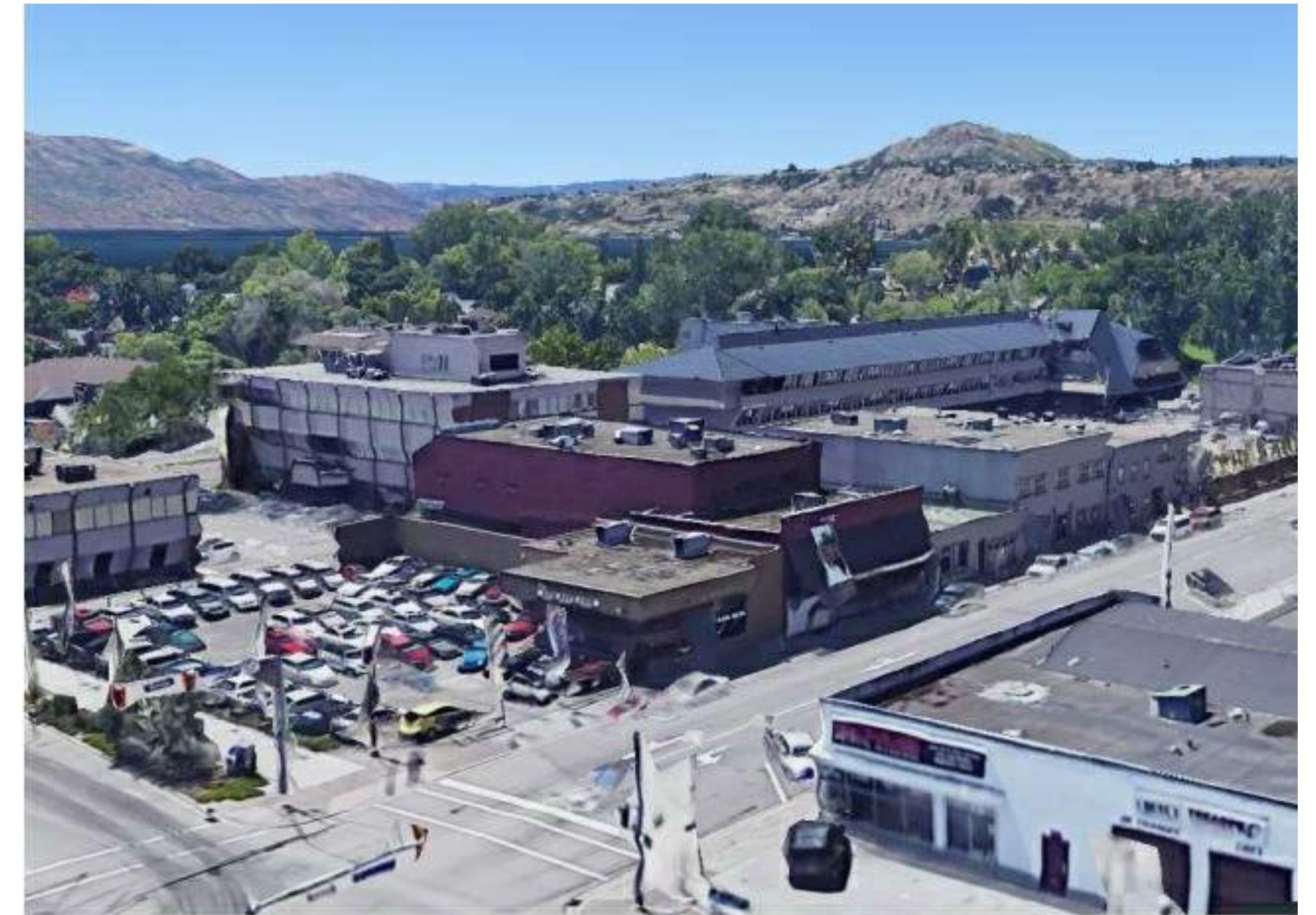
3 - VIEW FROM NORTH WEST WATER ST / VIEW FROM WEST WATER ST
