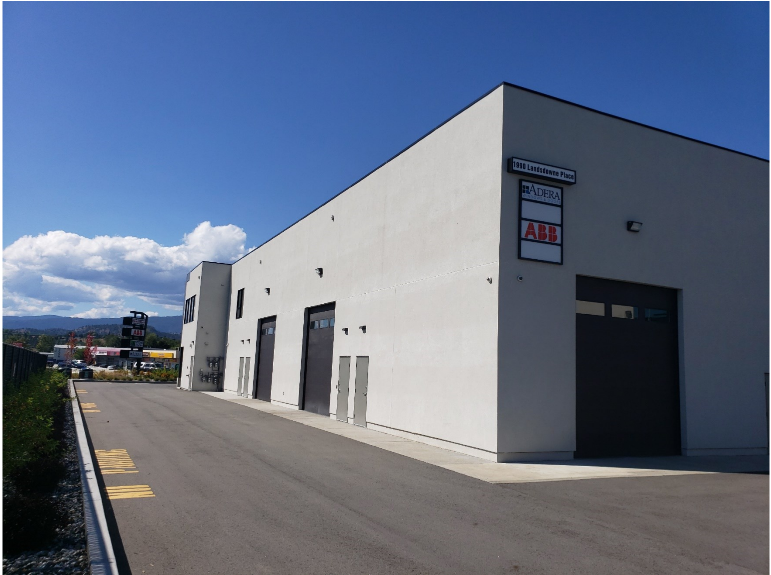
Side of Building
