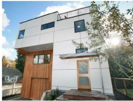
HARDIE REVEAL PANEL (SMOOTH) W/ PAINTED EXP. FASTENERS; COLOR ARCTIC WHITE (#2)
