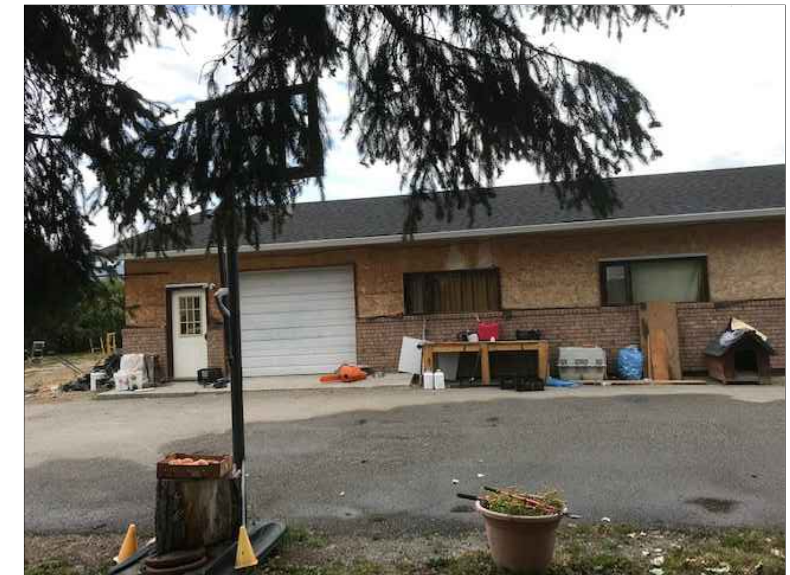
3 A2 REAR VIEW OF STORAGE END
