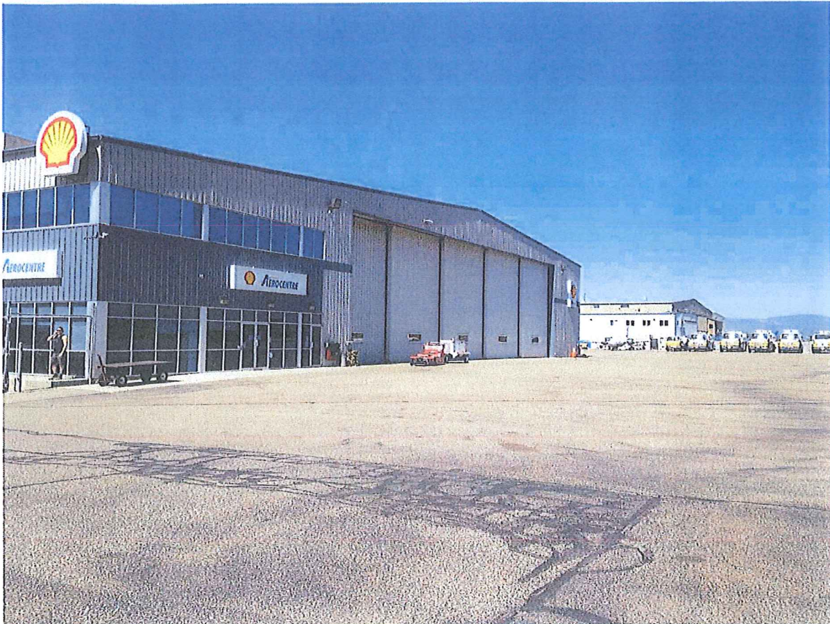
This facility houses YLW's current fueling operations. This photo was taken from YLW's apron, looking North West. This facility is on the West side of the runway, North of the terminal.
