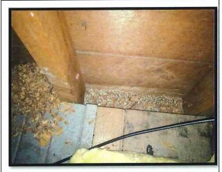
Vermiculite insulation present within the wall cavity of the east wall of the living room (Loc. 8) contains asbestos.
