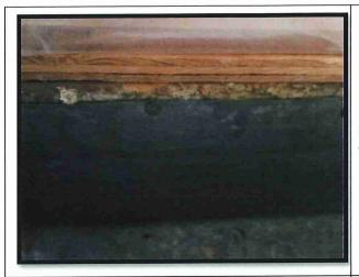
Duct wrap applied to floor registers throughout the top floor was found to contain asbestos.
