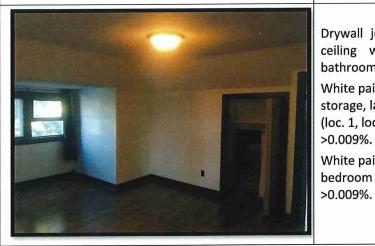
Drywall joint compound applied to drywall walls and ceiling within the landing, bedroom #3, storage, bathroom, bedroom #4 (loc. 9-13) contains asbestos.
