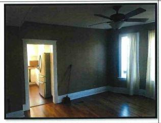
Brown paint applied to plaster within the dining room (loc. 2) has a lead content >0.009%.
