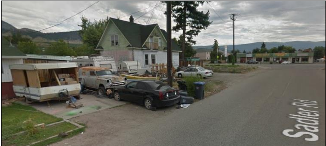
Fig. 2: Street view of 180 Hwy 33 E taken from the northwest, along Sadler Road. It is believed this is a similar view of the house as illustrated in the 1906 historical photograph featured in Fig. 7 below. (Source: Google Street View, 2017)
