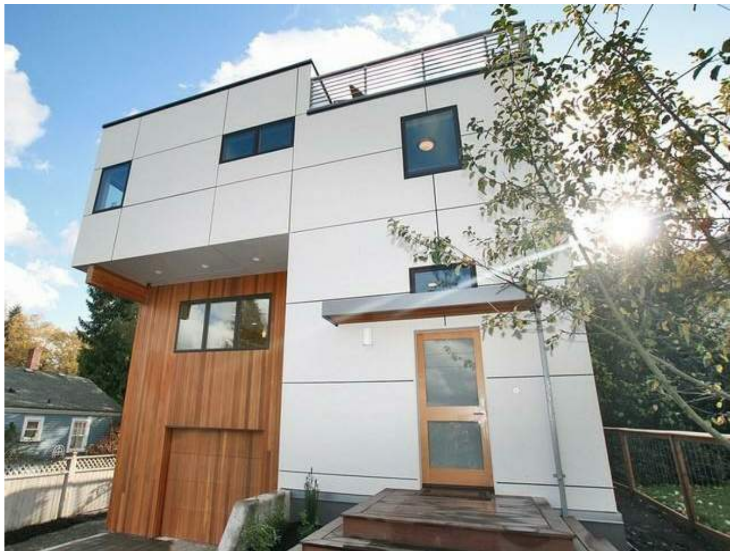
HARDIE REVEAL PANEL (SMOOTH) W/ EASY TRIM REVEAL & PAINTED EXP. FASTENERS; COLOR PURE WHITE SW 7005 (#2)
