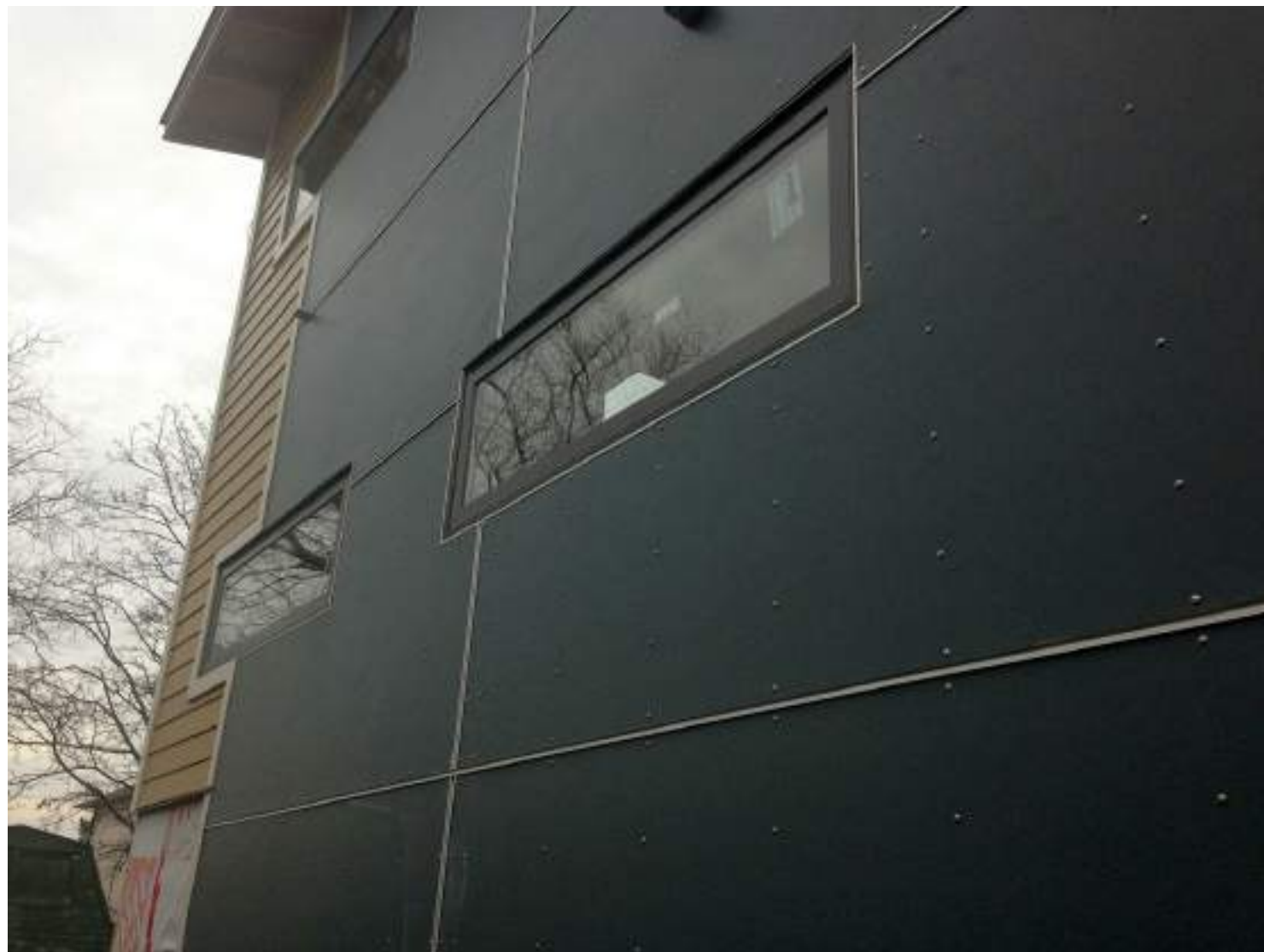
HARDIE REVEAL PANEL (SMOOTH) W/ PREFIN. ALU BREAK SHAPE (COLOR TO MATCH) & PAINTED EXP. FASTENERS; COLOR CAVIAR SW 6990 (#1)
