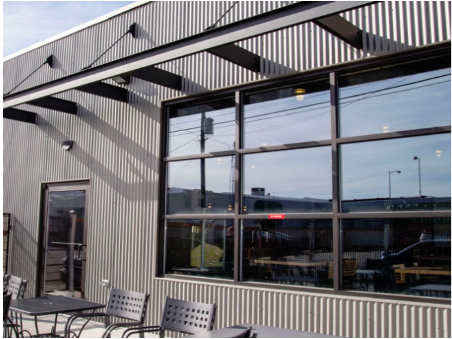
HORIZONTAL (#2) OR VERTICAL (#3) PROFILED METAL CLADDING - GALVANISED
