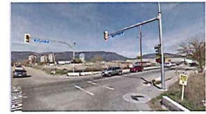
P1: Existing Site view from corner of Clement Ave and Richter St
