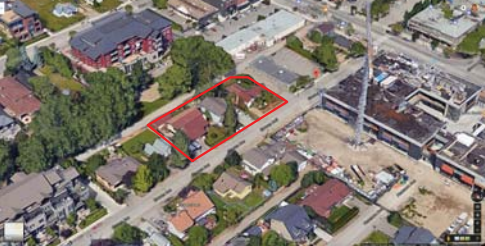
SOUTH-WEST AERIAL VIEW
