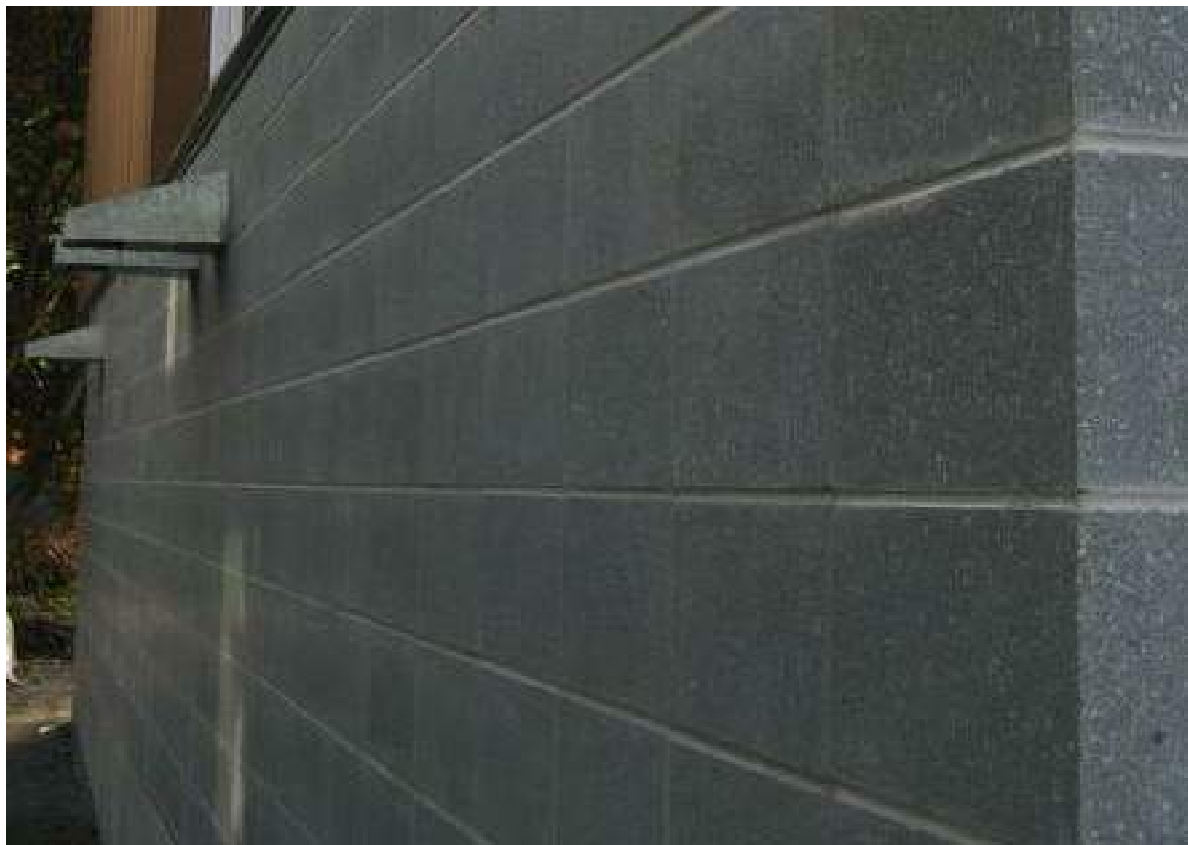
PAINTED TO SUIT (RICH ESPRESSO) STACK BOND BLOCK PATIO PRIVACY WALL (#11)
