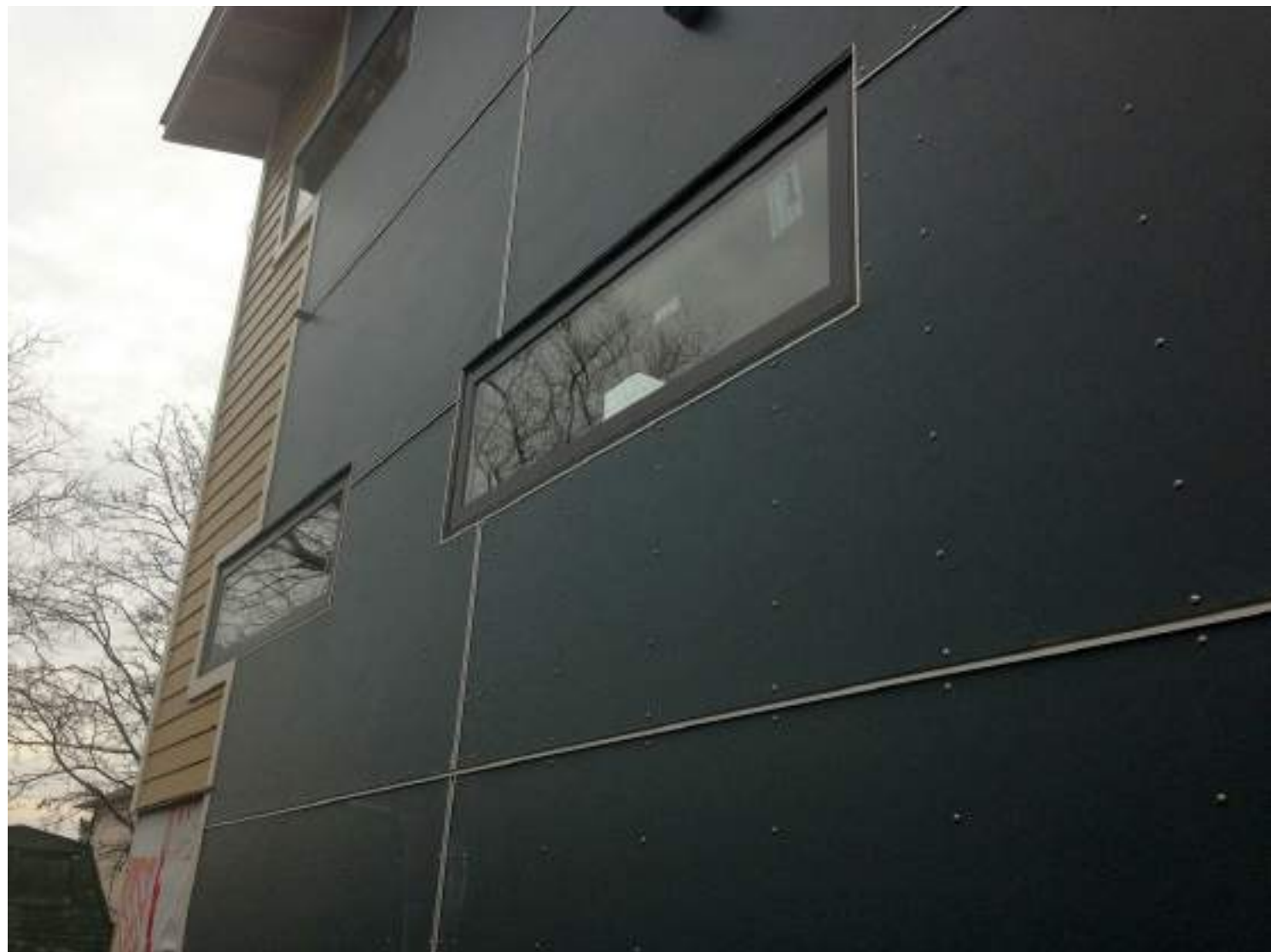
HARDIE REVEAL PANEL (SMOOTH) W/ PAINTED EXP. FASTENERS; COLOR RICH ESPRESSO (#1)
