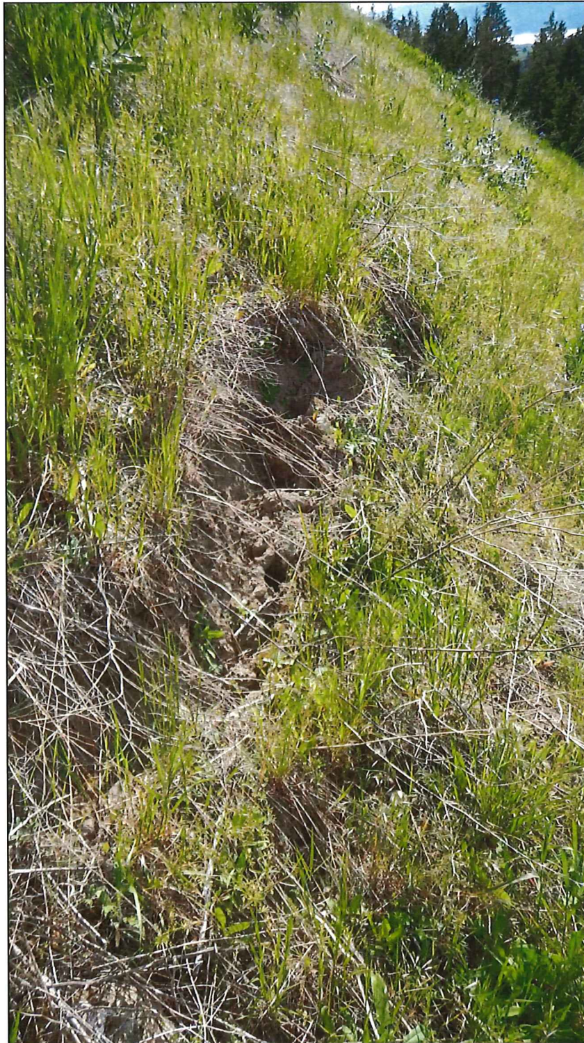
Photo 3: Looking at the tension crack in the fill slope at the rear of one of the un-developed lots to the southwest of the pump station.
