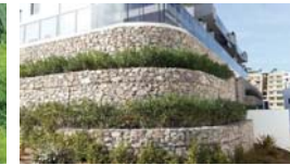
GABION RETAINING WALL WITH TERRACE PLANTING
