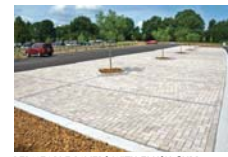
PERMEABLE PAVERS WITH FLUSH CURB
