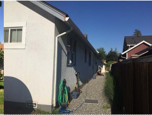
422 Cadder Ave.-Rear View
