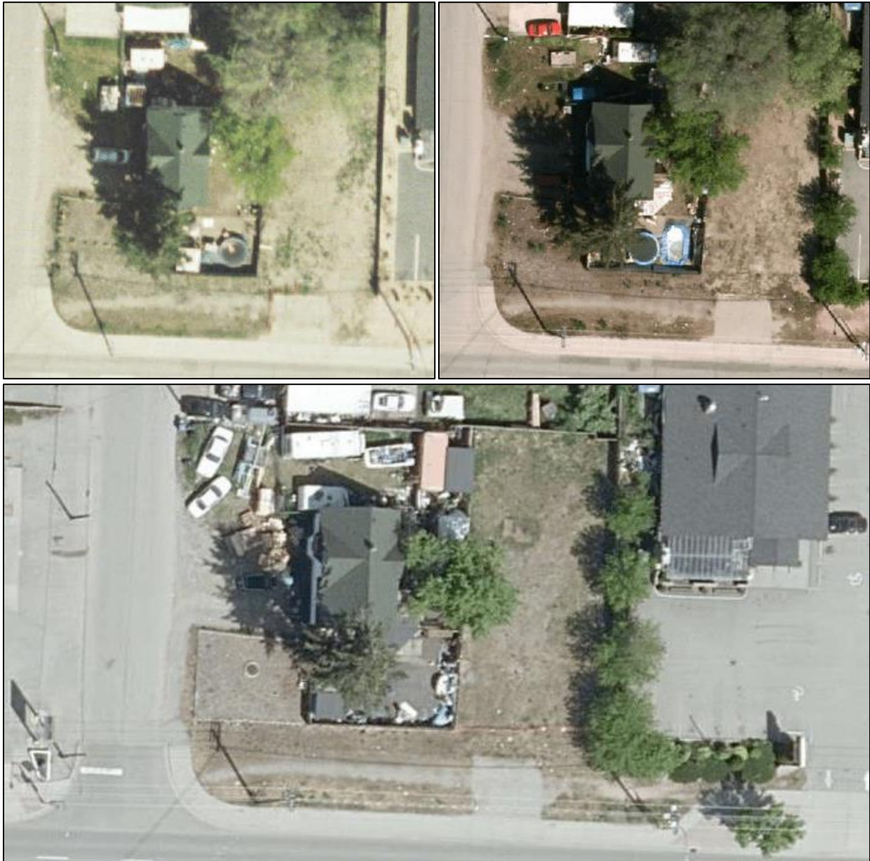
Figs. 14, 15 and 16: Comparative aerial views of 180 Hwy 33 E, 2006 (top left), 2012 (top right) and 2017 (bottom). (Source: City of Kelowna Map Viewer 2006, 2012 and 2017).
