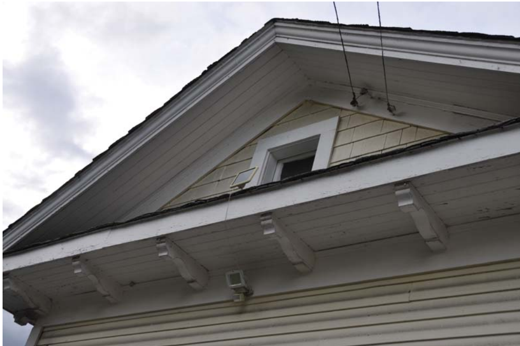
Photo 6. View of detail in the eaves, including corbels.
