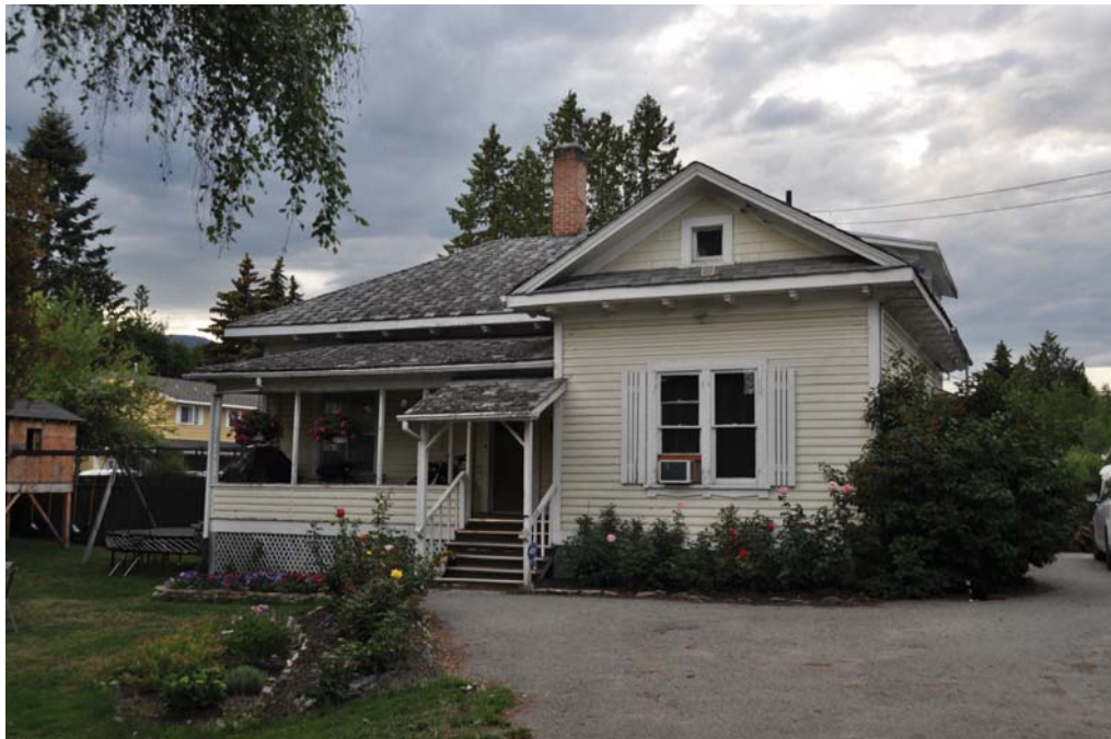
Photo 2. View of Smith residence from south (Cadder Avenue).
