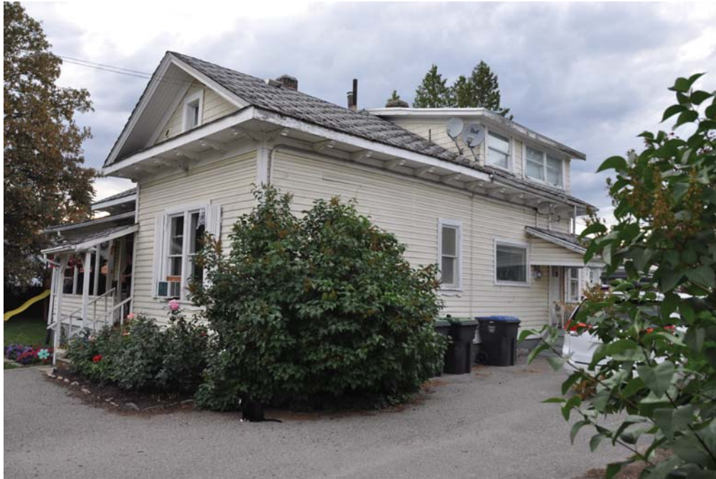
Photo 3. View of Smith residence from southeast (Cadder Avenue).
