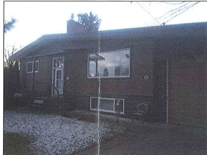
1 A1 STREET VIEW OF RESIDENCE
