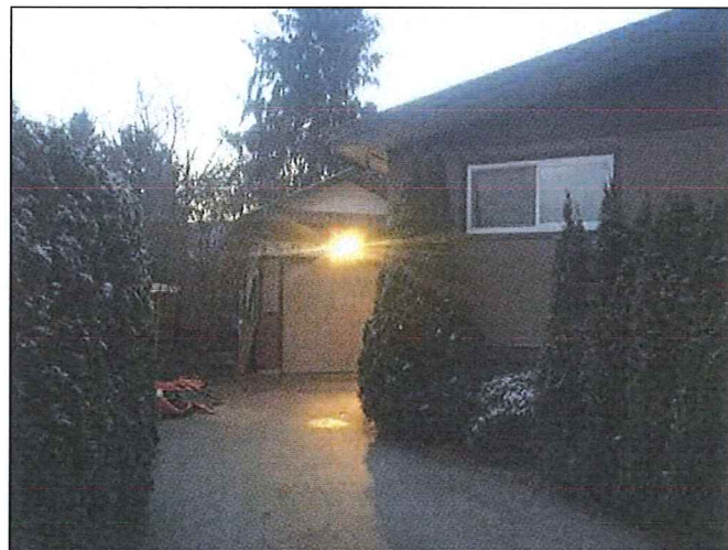
2 A1 STREET VIEW OF EXISTING GARAGE
