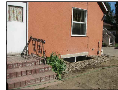
VIEW OF WEST ELEVATION
