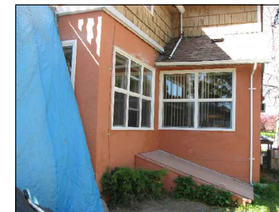
VIEW OF SOUTH ELEVATION
