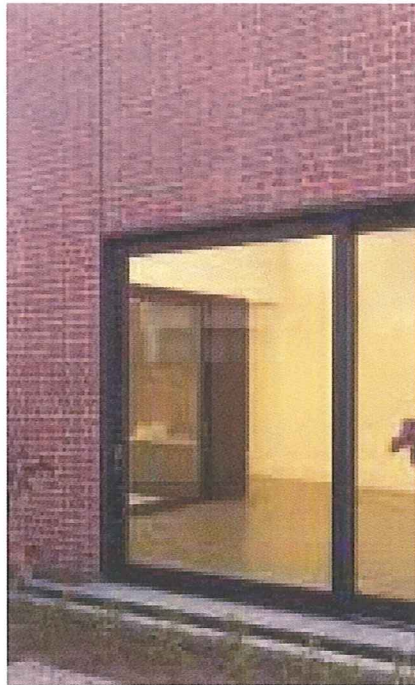
BRICK FINISH WITH DARK WINDOW FRAME
