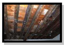
When the kitchen ceiling was removed, a four-inch thick concrete slab was revealed, installed no doubt, over a hundred years ago to keep the original cast iron tub from crashing through the floor boards into the kitchen below.
