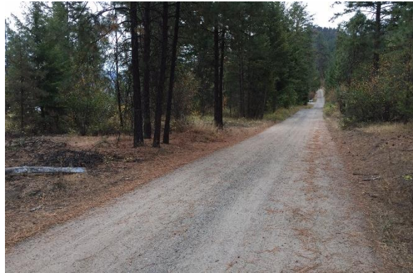
Current Condition of Shanks Road – South View
