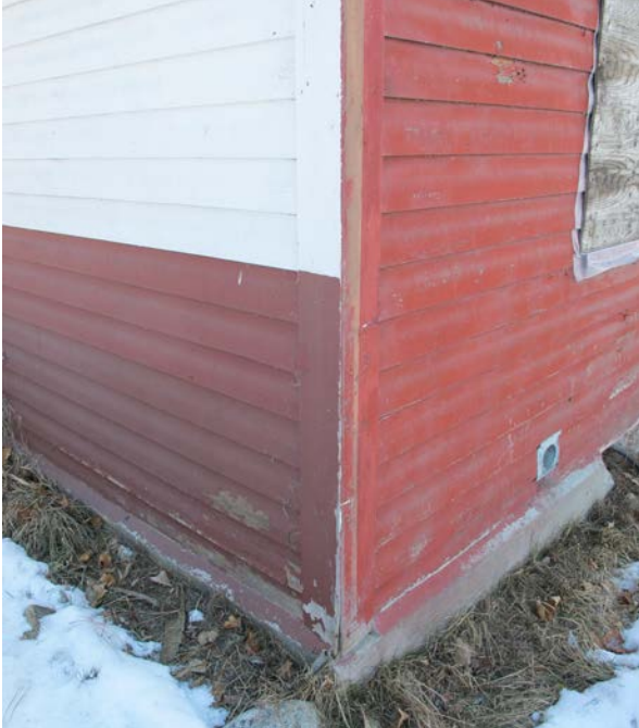
Northeast corner condition of the existing, original exterior walls of the Surtees Barn, showing unsympathetic paint finish.
