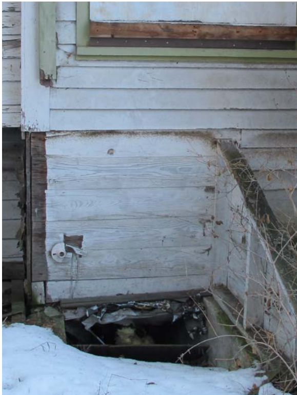
Portion of rear elevation showing opening to unoccupied partial basement, with exposed cast-in-place concrete foundation walls.
