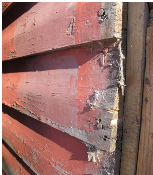
Photos showing typical deteriorated condition of exterior wall cladding, as well as roof soffit and corner board trims.
