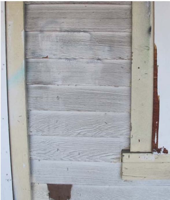
Photos showing original exterior walls with original materials interfaced with later rehabilitation with inappropriate detailing; at historic front facade between door and window opening (bottom left), and at south elevation and return wall of later addition (bottom right).
