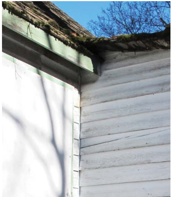
Photos showing original exterior walls with original materials interfaced with later rehabilitation with inappropriate detailing; at historic front facade between door and window opening (bottom left), and at south elevation and return wall of later addition (bottom right).
